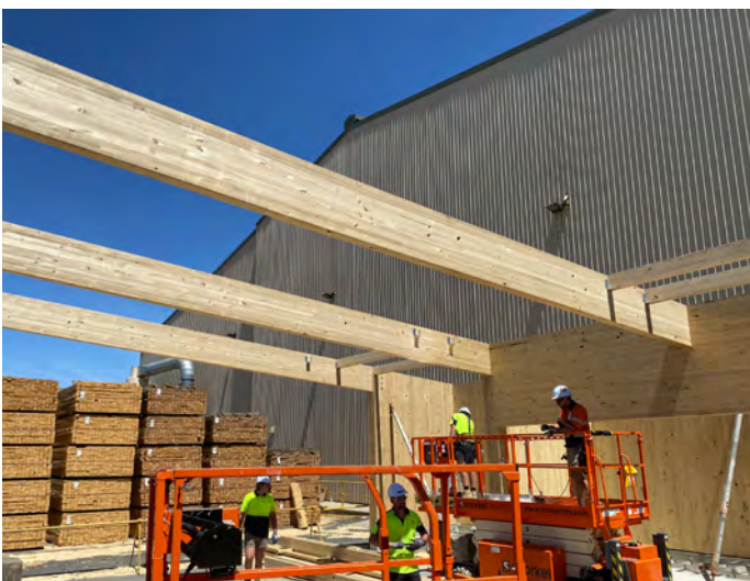
NeXTimber GLT beams on display during construction.
