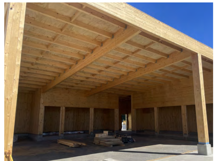
The charging station with NeXTimber CLT roof panels installed.
