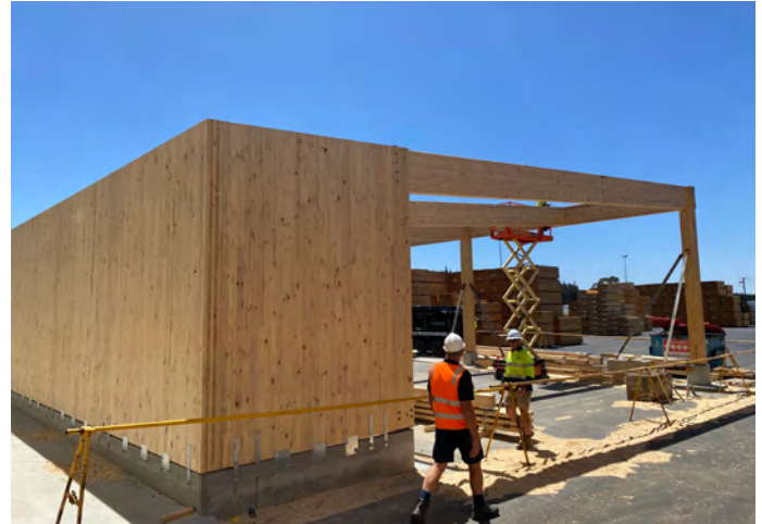
The charging station under construction using NeXTimber CLT & GLT.
