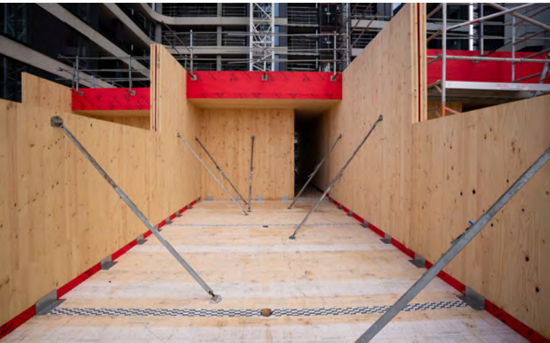
Installation of CLT panels taking place.
