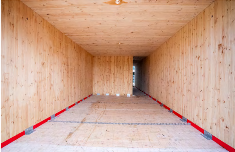
Another internal view of our installed CLT panels.
